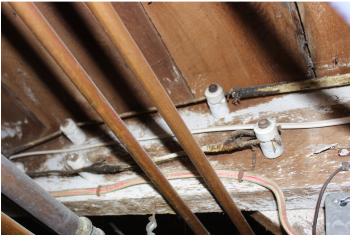
Electrical Terminated wires (knob and tube)
