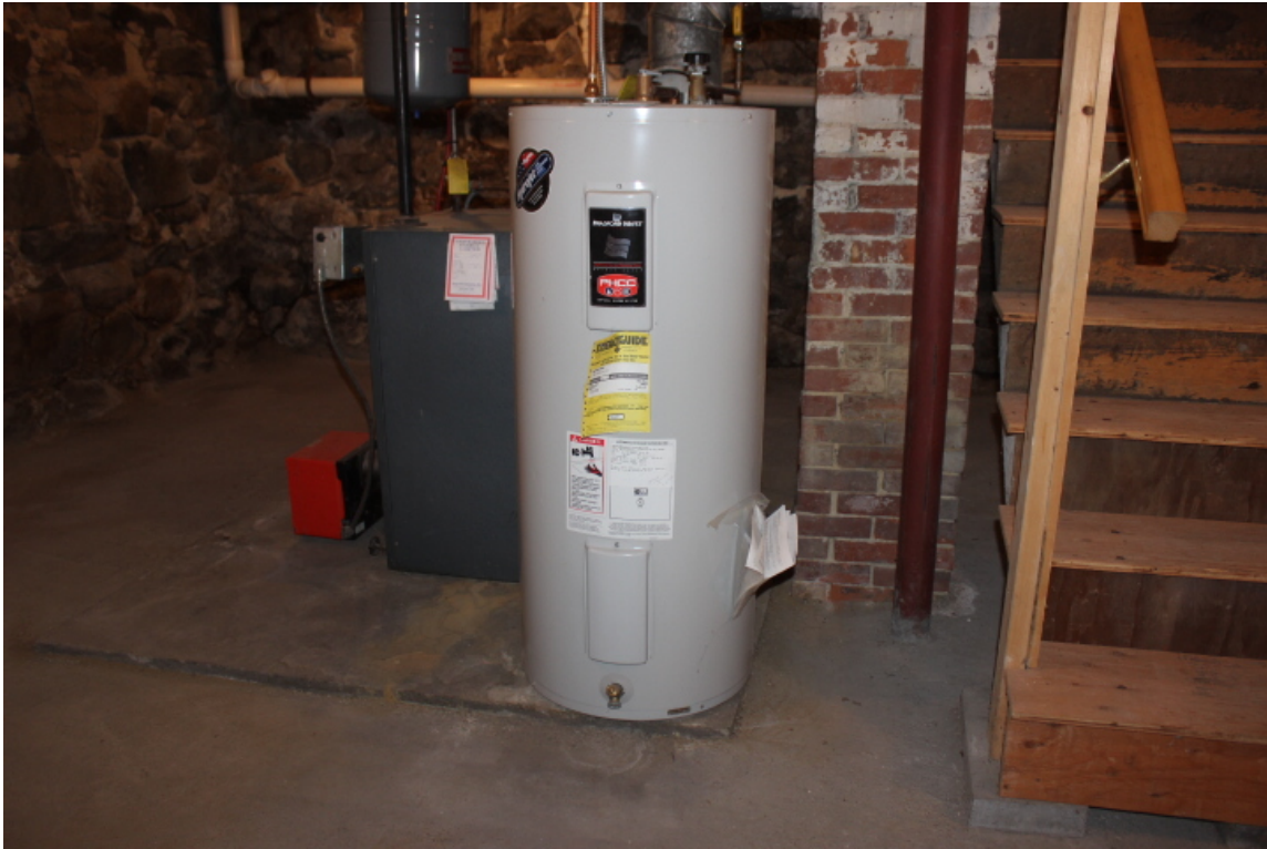
Plumbing Water Heater
