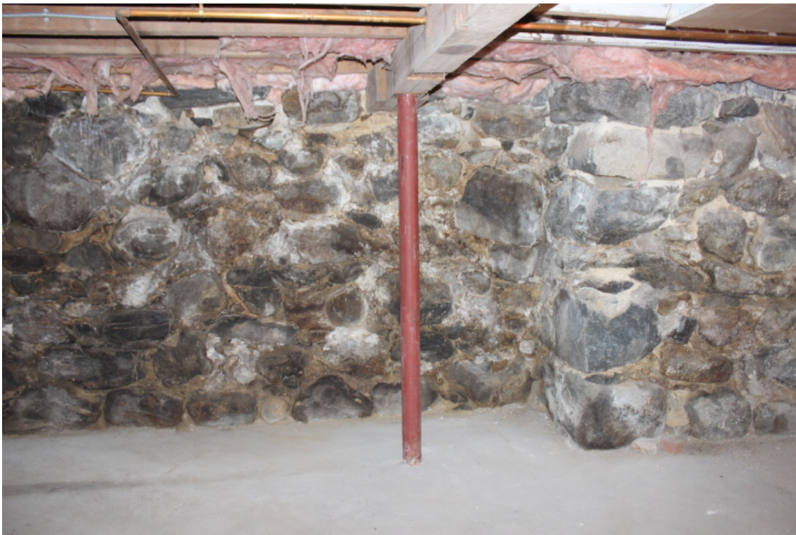
Foundation Wall dampness (rear)
