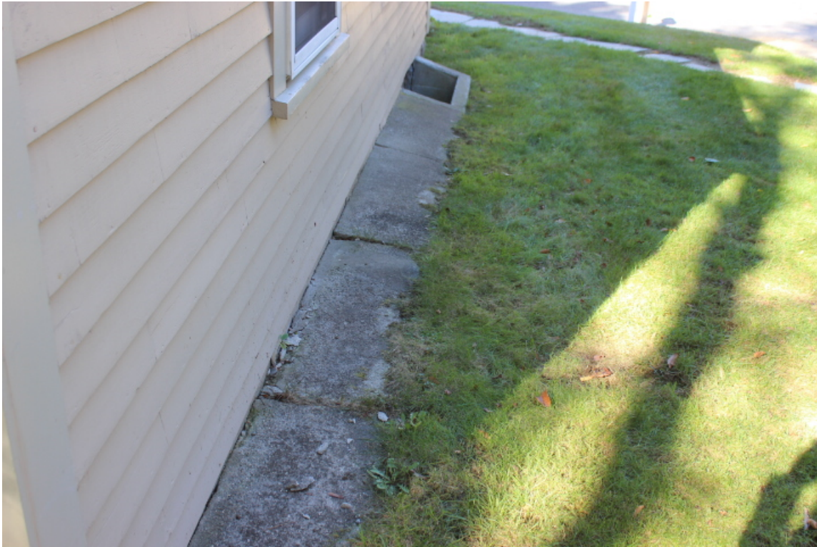
Grounds & Drainage Soil elevated against house (wood surface)
