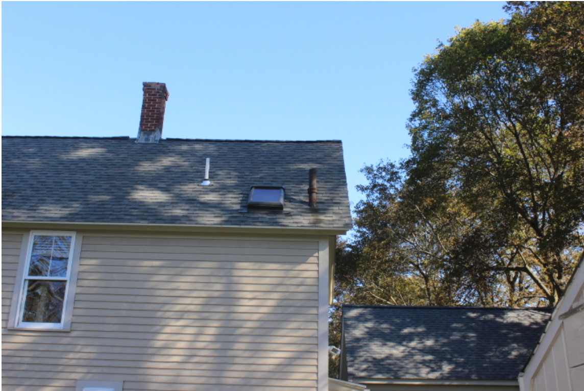
Roof Roof and chimney
