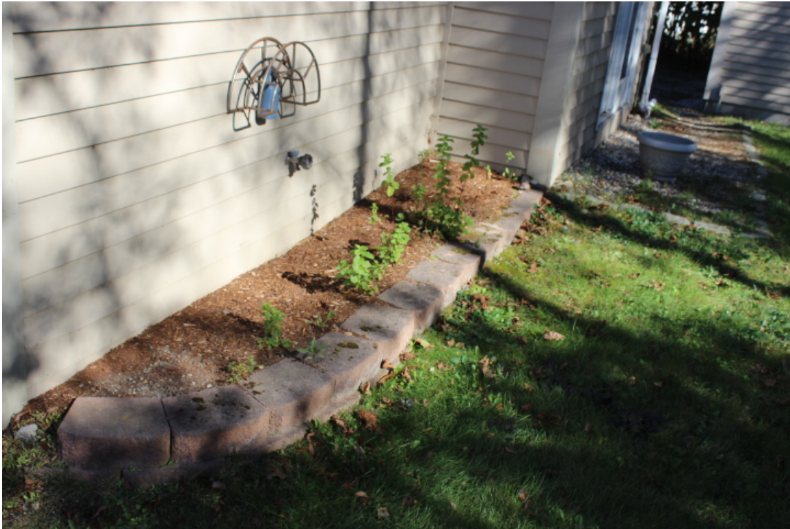
Grounds & Drainage Soil elevated at wall sill (cause for concern)
