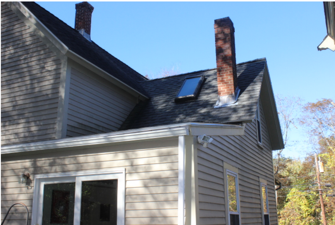
Roof Roof & Chimneys
