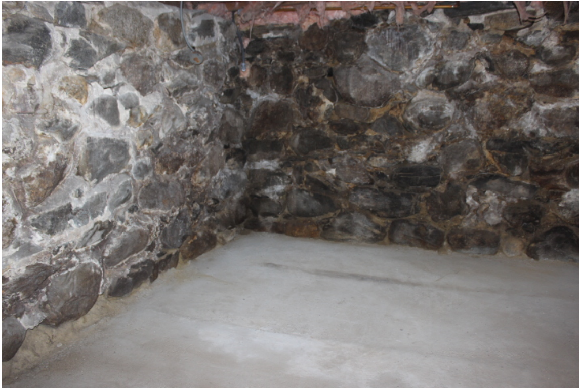
Foundation Dampness at rear wall
