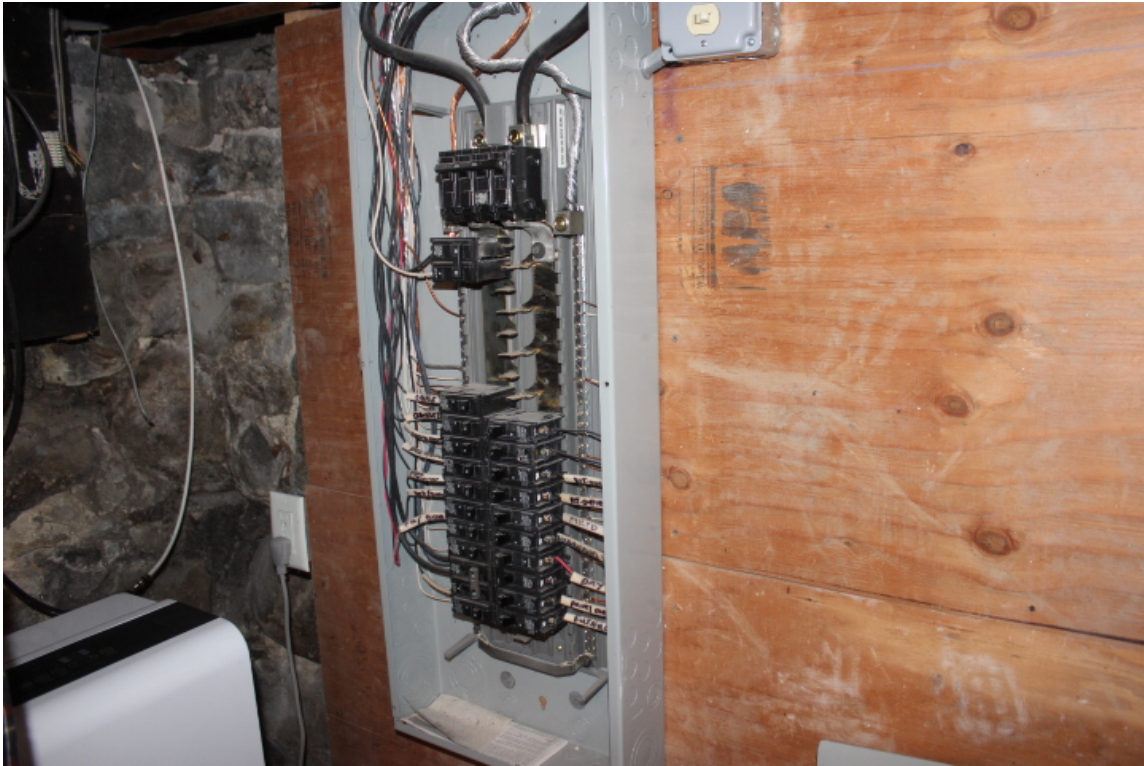
Electrical Main electric panel
