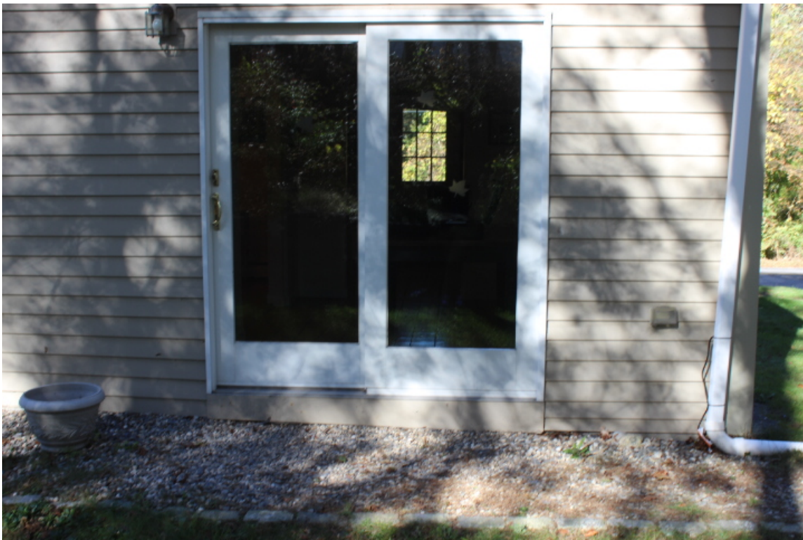
Grounds & Drainage Soil contacts wood siding (insect or decay is possible)
